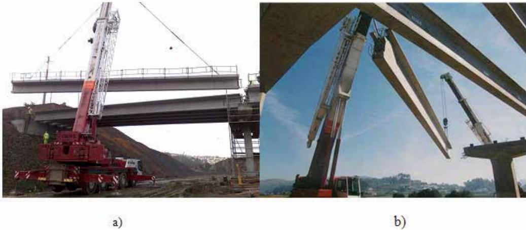
Figure 6. Placing of precast beams on the pillars (Leonhardt, 1982).
