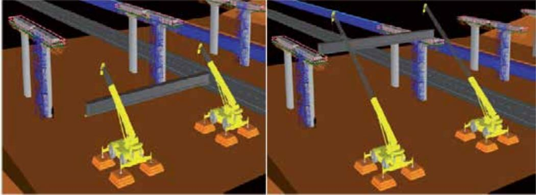
**Figure 13.** Prefabricated beams raised by two cranes.
