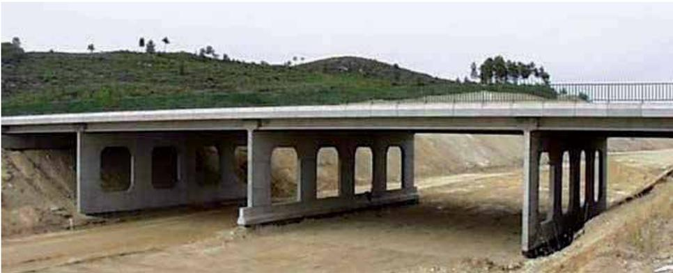
**Figure 4.** Overpass on A23 performed with prefabrication (Juntas, 2013)
