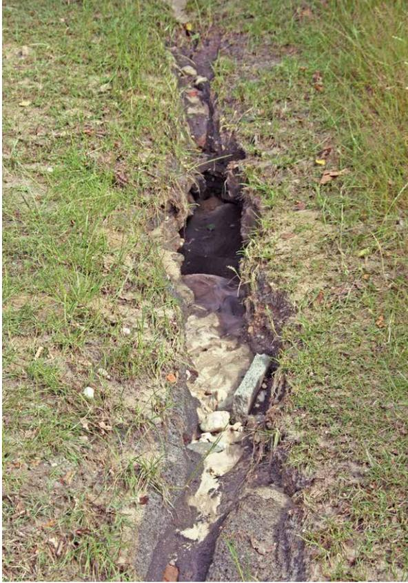
**Fig. 5.3:** Eroded ditch in the road following heavy rain fall in July 2009.
