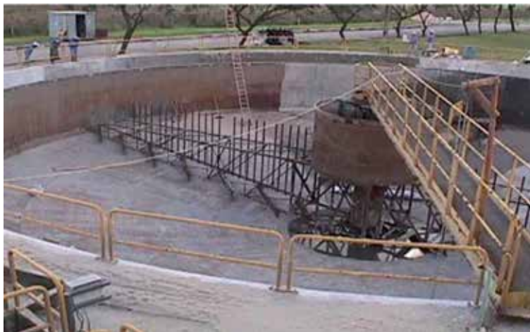
Figure 1. Sludge densifier by gravity. WWTP-Sabesp, São Paulo, Brazil (source: the author).
