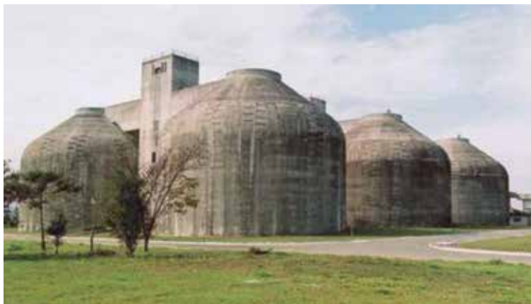
Figure 2. Anaerobic digester. WWTP-Sabesp, São Paulo, Brazil (source: the author).
