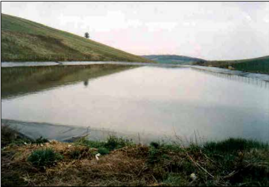
Picture 5. Large lagoon for storing digested pig slurry
